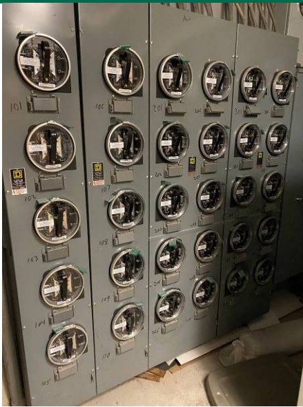
Owner Provided Interior Photo
