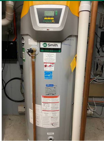
Owner Provided Interior Photo
